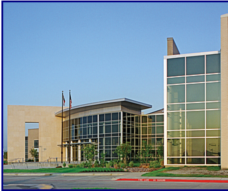
Figure 5 LaGrone Advanced Technology Center
